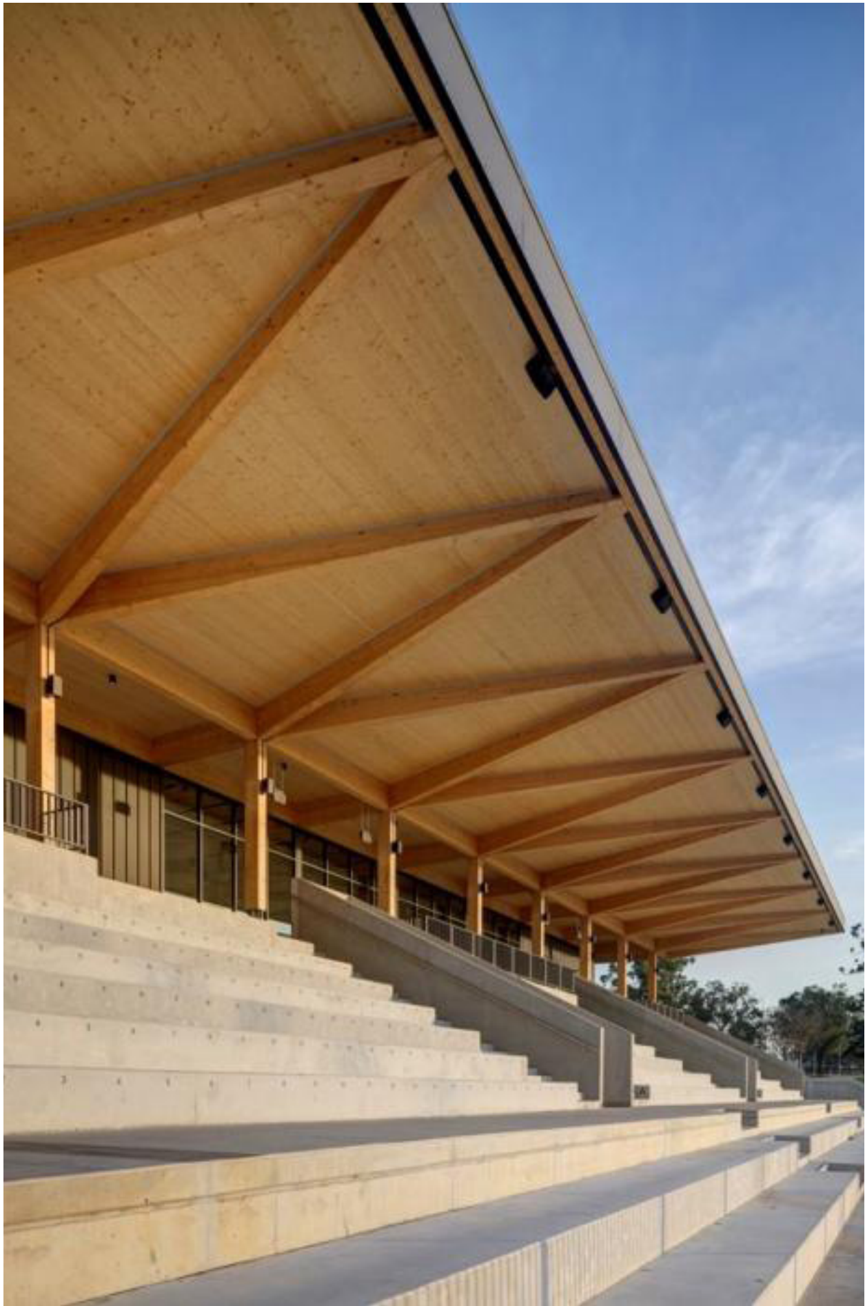
Eric Tweedale Stadium, Sydney, dwp / Northrop, www.northrop.com.au
